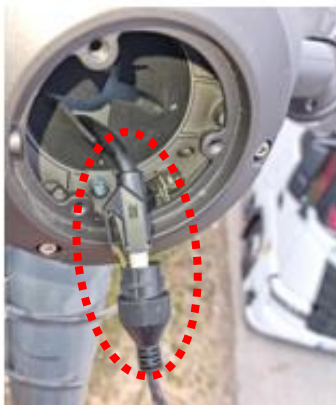
[Gasket & butyl tape missing]
